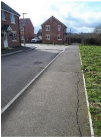
Figure 3 – Footway on Site Frontage
